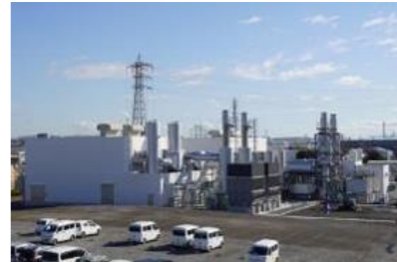
Completion of expansion work on in-house power plant
