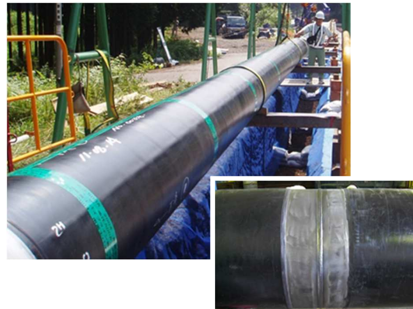
Steel Pipe Welds Resistant to Ground Tremors and Liquefaction
